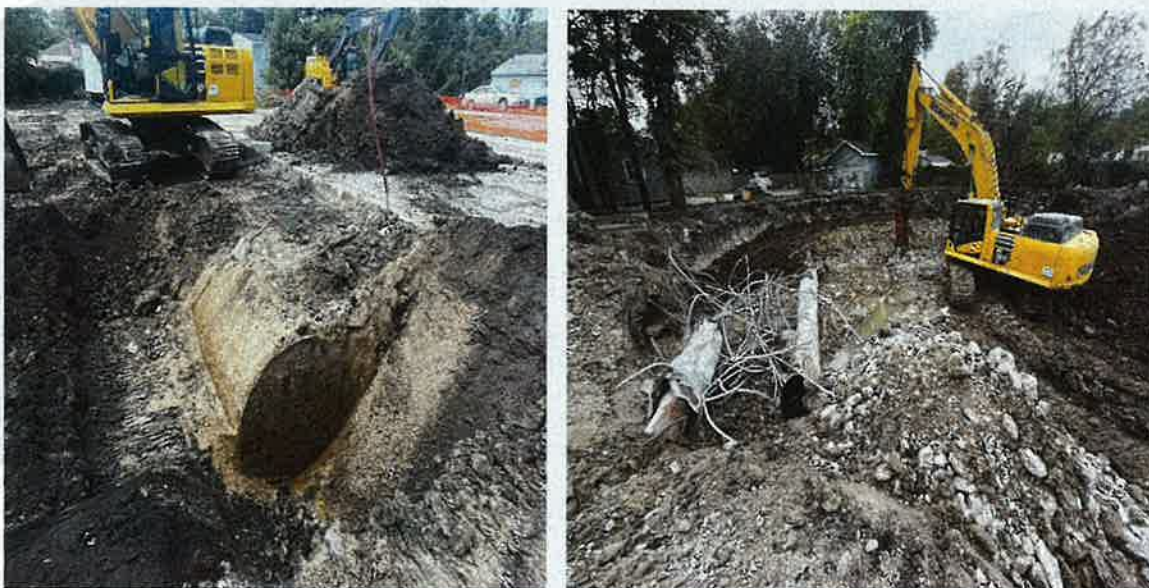
Contaminated Soil Tower #3
