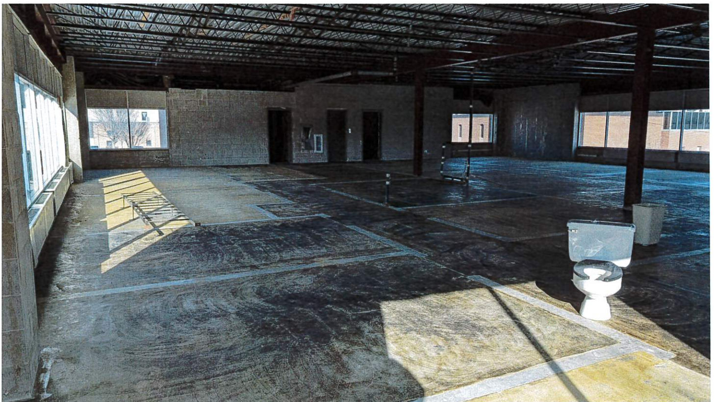
Images of interior after asbestos abatement
